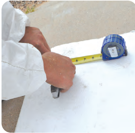
2. Cut blocking material to fit
