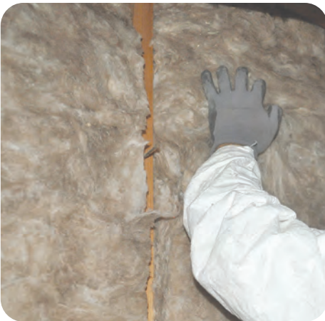
3. Install batts with minimal compression
