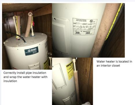
Photos of work to be performed on DWH, along with some example pictures of typical work performed.
