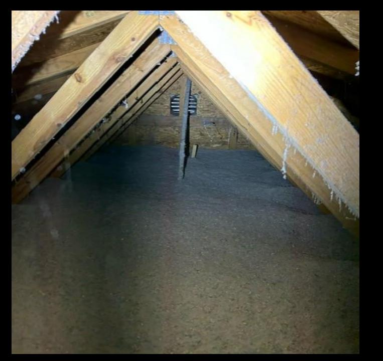
Depth markers: 1 depth marker should be installed for every 300 square feet of attic space.
