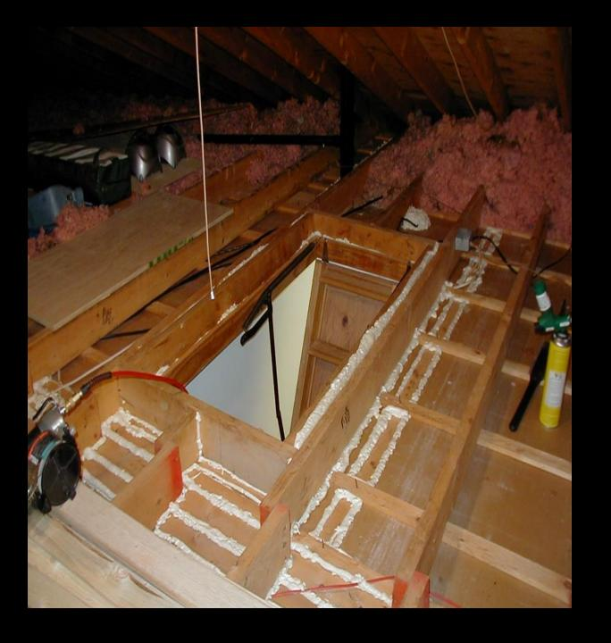
All penetrations, including top plates, should be air sealed before insulation is added.
