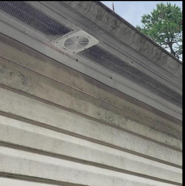
Proper roof ventilation will have a balance between air intake (at or near your soffits) and air exhaust (at or near your roof ridge). A minimum of 1 square foot Net Free Area of attic ventilation (evenly split between intake and exhaust) for every 300 square feet of attic floor space.
