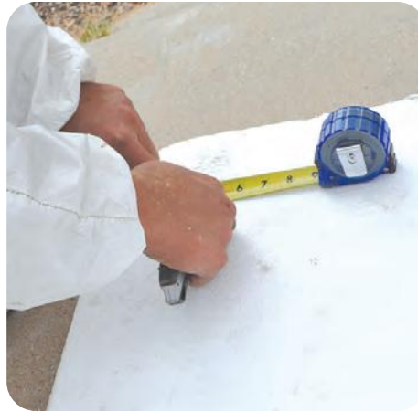
2. Cut blocking material to fit
