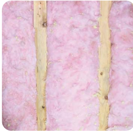
2. Cut batts for exact fit
