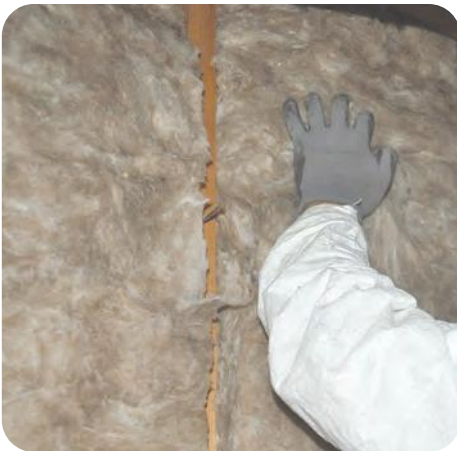
3. Install batts with minimal compression
